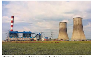
Nabha Power, a coal-fired supercritical power plant, operates two units, each generating 700 MW.
